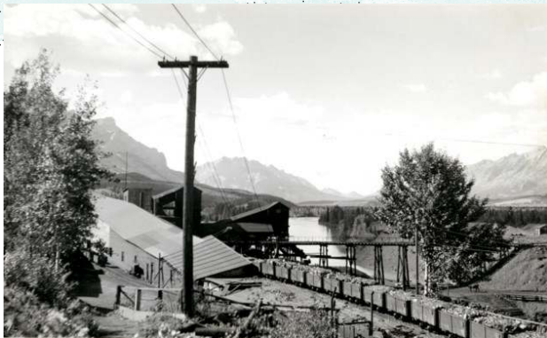
The No. 2 Mine looking north towards the tipple, 1956. CMAGS 2008.013.010.001
